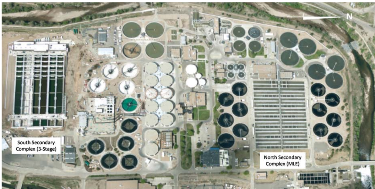
Figure 1: RWHTF Aerial: North and South Treatment Plants
